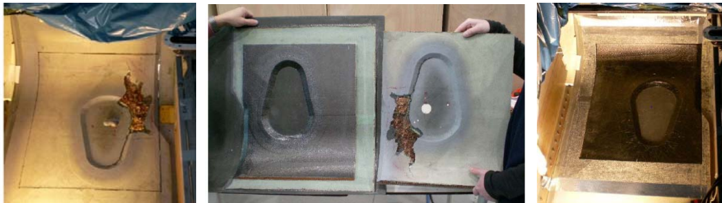
Figure 5-1: Cut-Out, Prepared Inlay, Fitted Inlay
